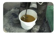
Make sure the resin container is secure (between your feet) before you start mixing.
