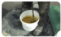
The Part A component resin should be mixed briefly (10-20secs) using a slow speed, high torque, helical blade mixer. Accelerator/Catalyst should be added at this stage if needed – see Accelerator/Catalyst guidelines for details.
