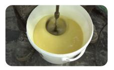
Part B component resin should then be added and mixed thoroughly at slow speed for a minimum of 60 seconds until uniform.
